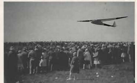
Fig 11. The Wien being bungy launched. Normally four to six runners would pull on each end of the rope.
